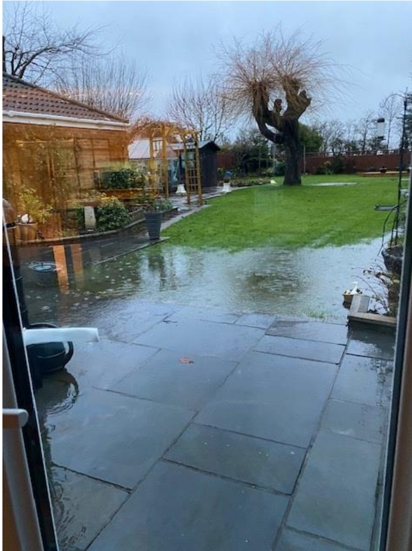
(Figure 11 – Flooding in the rear garden at Property C, as provided by the resident; facing north)
