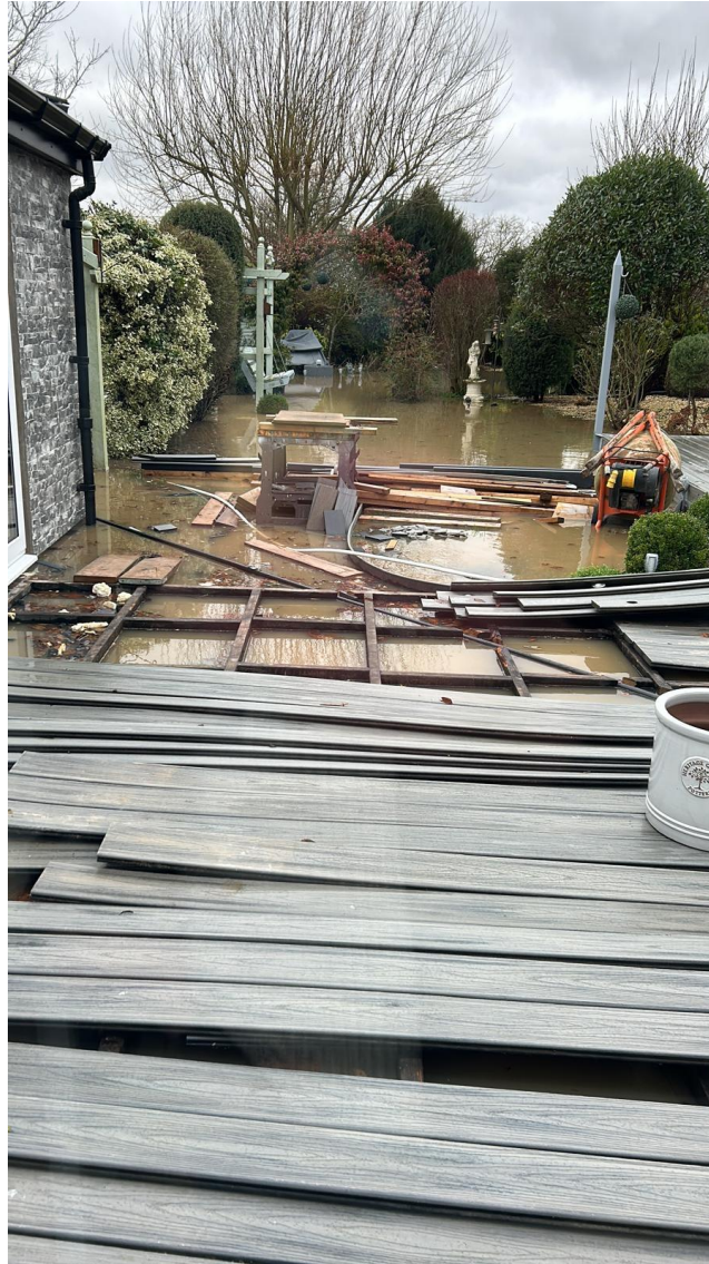
(Figure 16 – Flooding in the rear garden at Property D, as provided by the resident; facing north)
