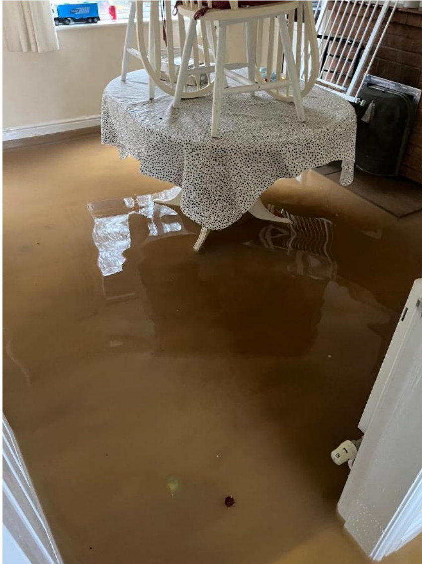
(Figure 10 – Internal flooding within Property A, as provided by the resident)
