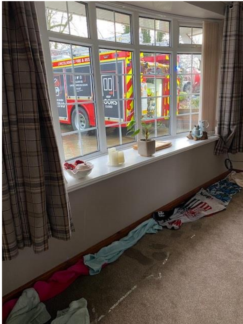
(Figure 13 – Seepage at Property C, as provided by the resident)
